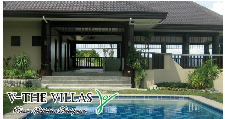
VILLAS DEL PUEBLO (BY V-THE VILLAS) TAAL BATANGAS COMPLETED 2012
