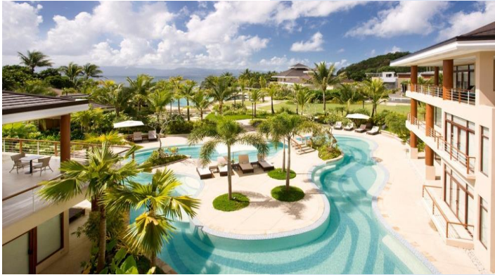
MISIMIS BAY (PLUMBING & POOL EQUIPMENTS) BICOL REGION COMPLETED 2009
