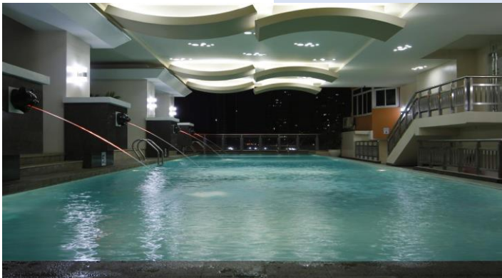
REGENCY GRAND SUITES (PLUMBING & POOL EQUIPMENTS) MANILA COMPLETED 2009
