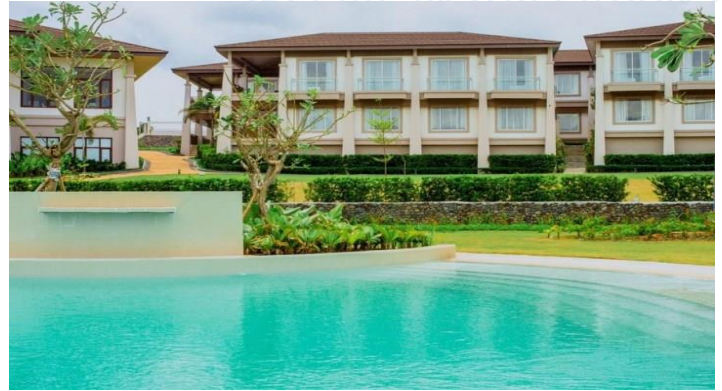
ACEA BAY (PLUMBING & POOL EQUIPMENTS) SUBIC COMPLETED 2012
